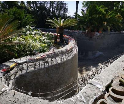
Gunite application and progress. Note the sand filled bags creating a temporary formwork and light steel mesh installed prior to gunite application.
