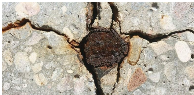
Fig. Example of negative effects of carbonation to reinforcing steel (Source: Reinforcement Corrosion and Structural Safety Group of the Eduardo Torroja Institute)
